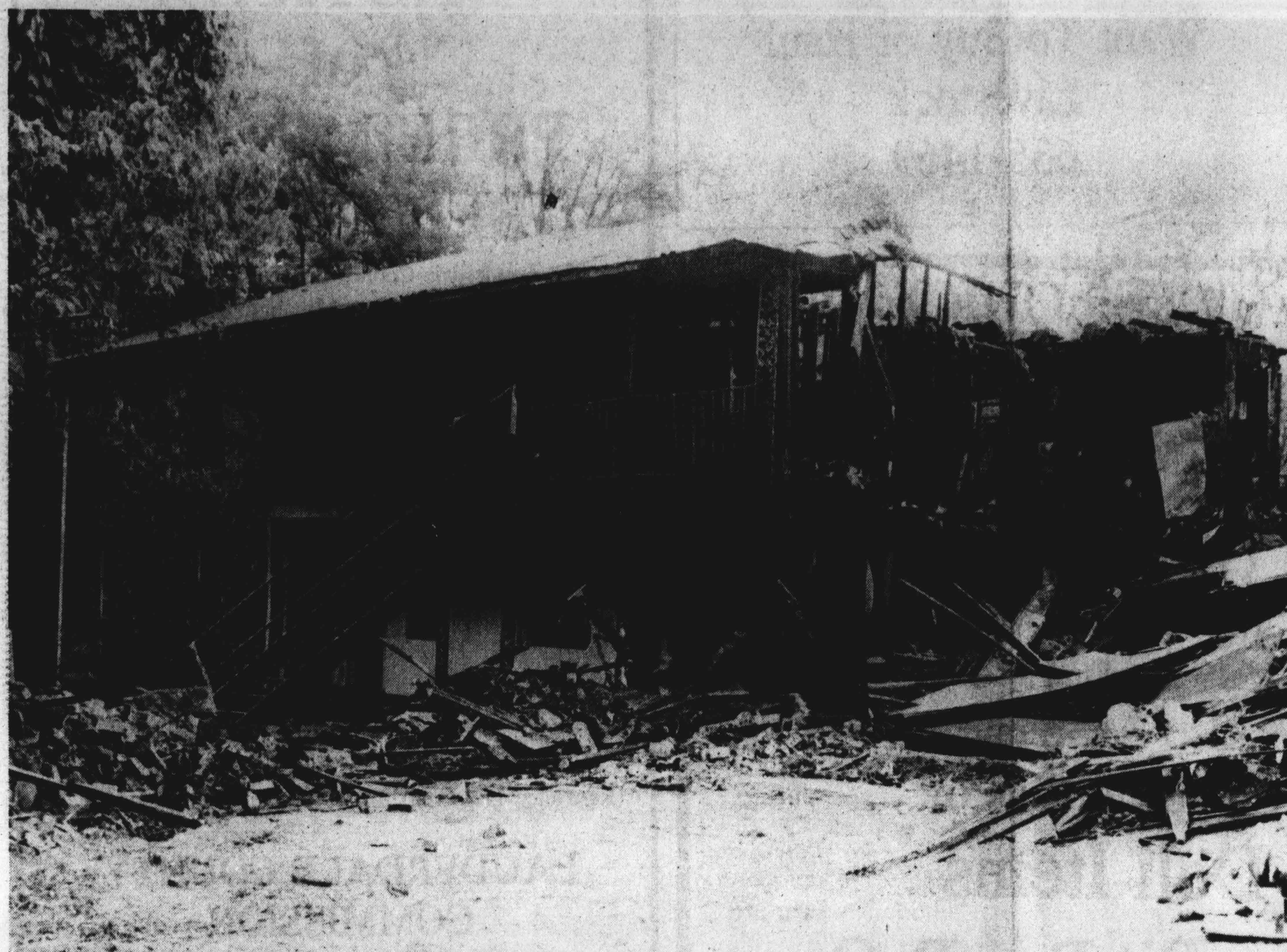
FATAL FLAMES heavily damaged the 8-unit Greenhill Apartments at 293 Gay in Ripley, owned by Albert Thornton, of Ripley, about 3 a.m. Sunday.
